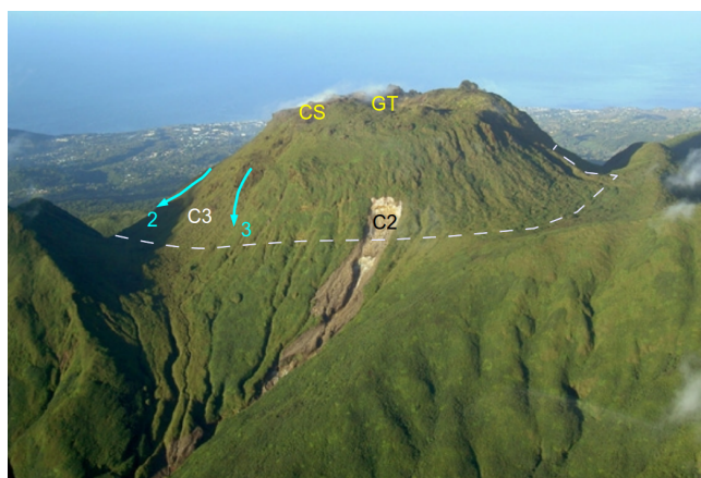
Figure 1. La Soufrière lava dome seen from North-East. The dashed line marks the Eastern segment of the electrode line shown in Fig. 2. The small landslide visible on the picture is located in front of the C2 conductive region of Fig. 8, and the blue arrows mark two lahars that occurred during the 1976 – 1977 crisis in front of the C3 conductive region (see also Figs 8 and 9). The CS and GT labels respectively point the South Crater and the Tarissan pit locations (green points in Fig. 2).
