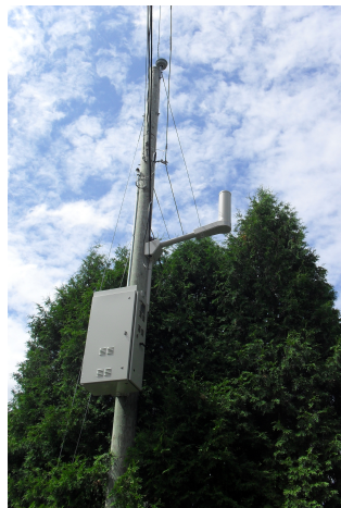
A distributed antenna port used in the Videotron 3G network in Montreal, Quebec (Source: Wikipedia).
