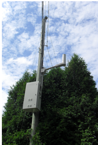
A distributed antenna port used in the Videotron 3G network in Montreal, Quebec (Source: Wikipedia).
