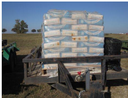
Bentonite Storage at Site
