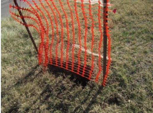
Locating Underground Utilities
