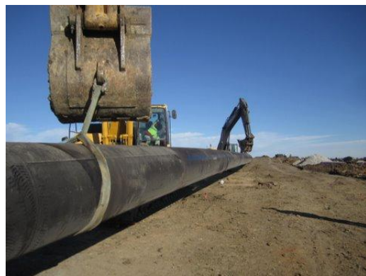
Hoisting Steel Pipe
