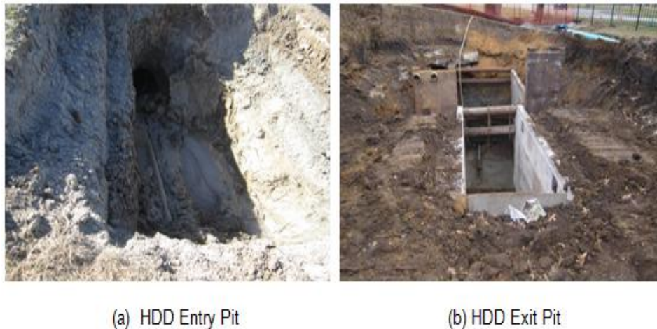
Figure 4.3 HDD Entry and Exit Pits
