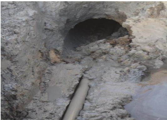
Prereaming/Reaming of Borehole
