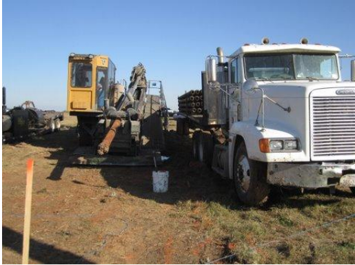
Start of Pilot Hole Drilling
