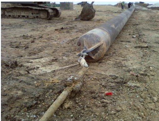
Connecting Steel Pipe
