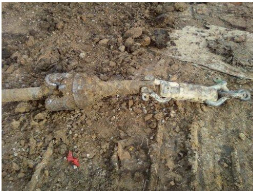
Connecting Swivel to Reamer
