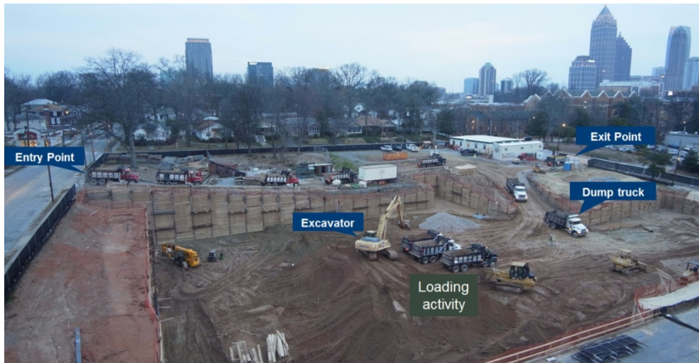
Figure 2. Overview of project under consideration
