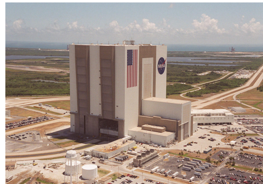
FIGURE 5: The Vehicle Assembly Building (VAB) was built for the Apollo program. The VAB was designed to house the assembly and final checkout of the 110-meter-tall Saturn V launch vehicle. One of the VAB’s most notable features is its 139-meter-high doors. It was also used for the assembly/stacking of the NASA Space shuttle. The VAB will be used for the assembly/stacking of the SLS and the MPCV. Photo courtesy of NASA.
