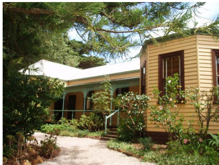
Figure 7.9 Churchill Island cottage
