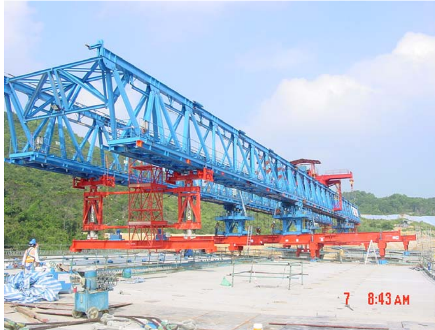
Figure 4.1: The Giant Gantry of the Stepping Girder for Erecting Precast Segments
