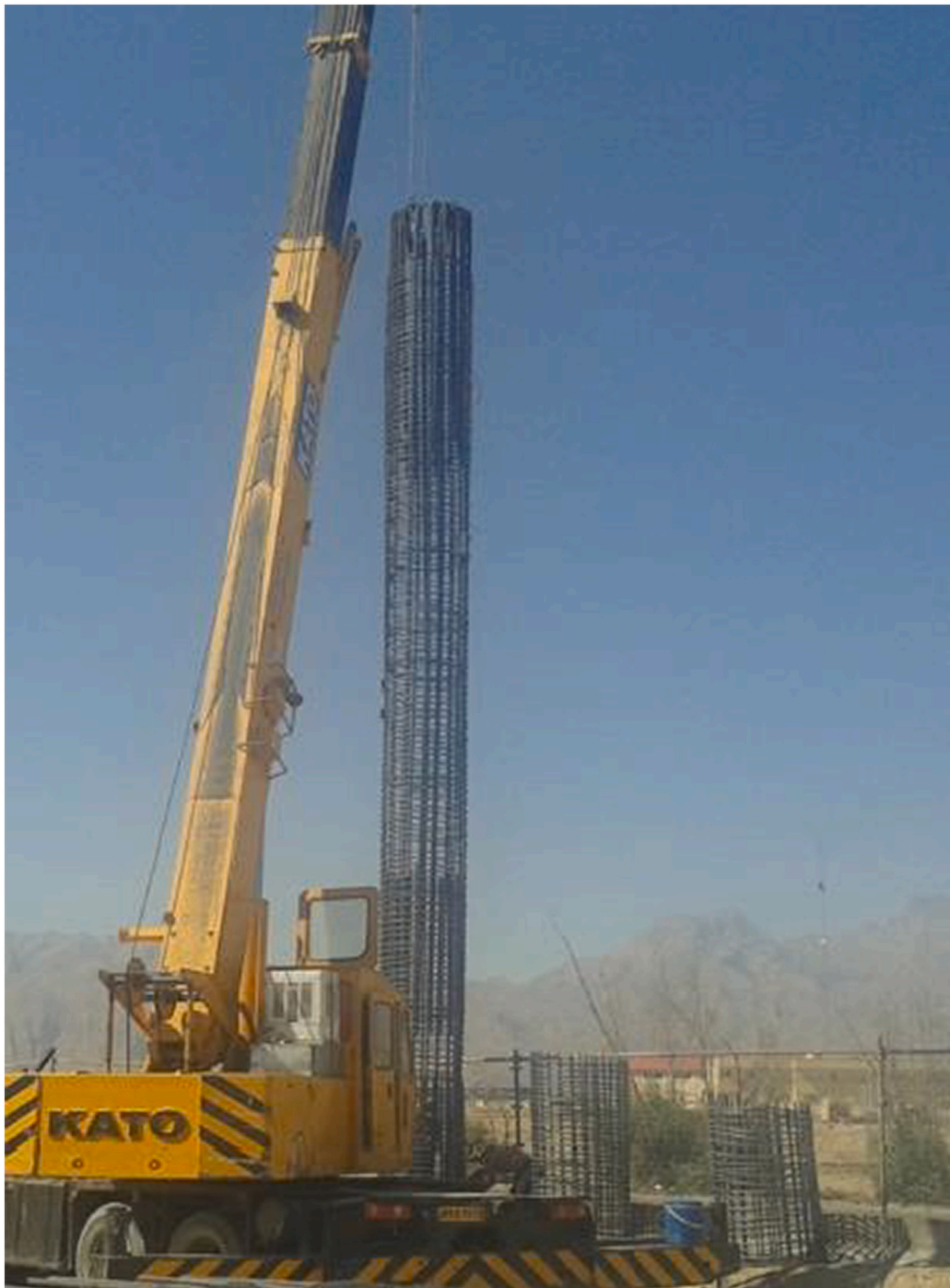
Fig. 9. Installation of a fabricated bar basket using a mobile crane.
