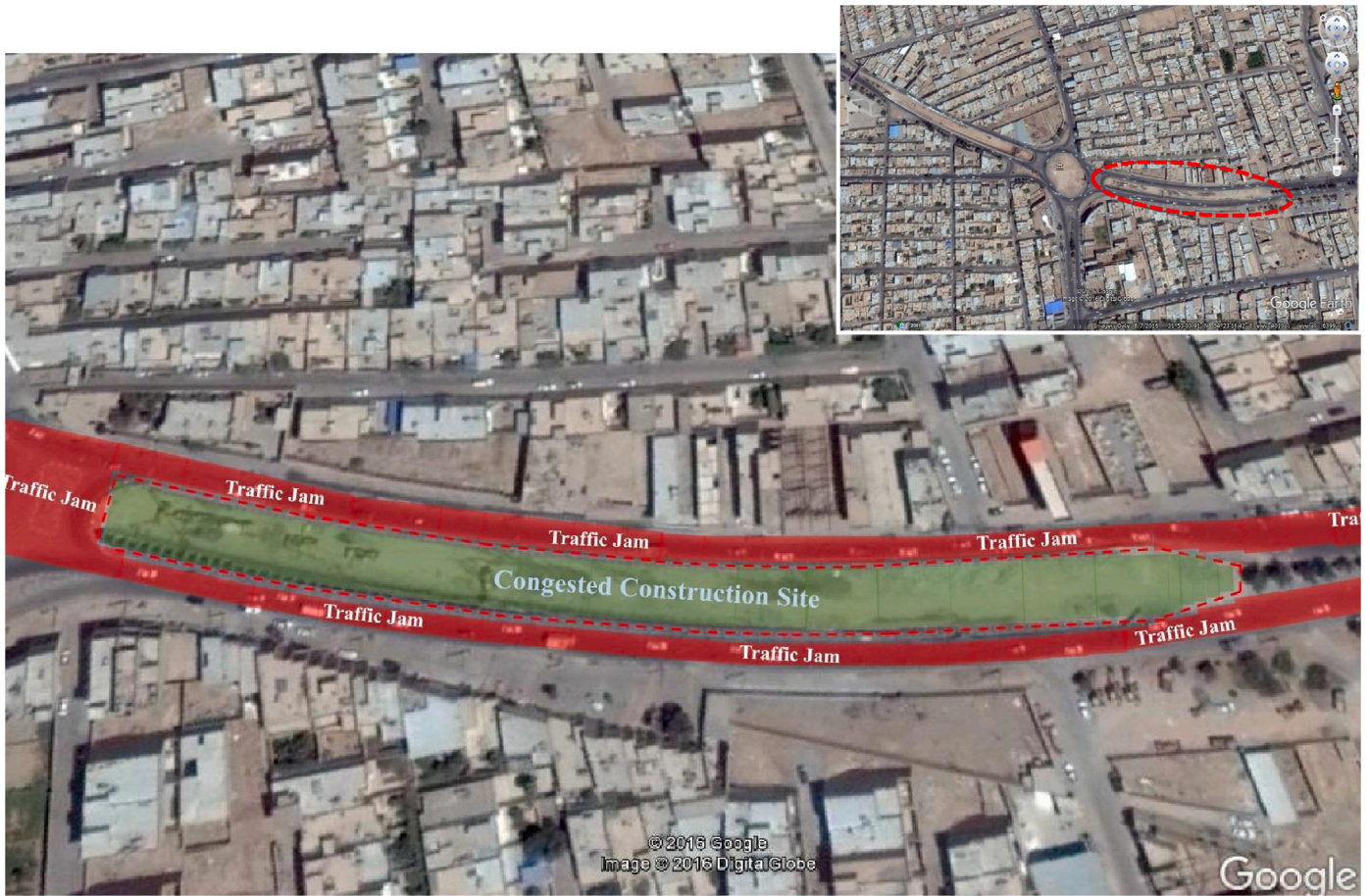
Fig. 7. Schematic plot and Google Earth aerial photo of the project (Yazd, Iran).
