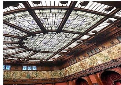
Figure 7. A sample of a glazed ceiling: the Velario in the Hall of Italian Parliament
