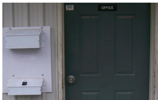
Fig. 2. Fingerprint scanner (lower white box) and video camera (upper white box) at Greeley, Ontario site.
